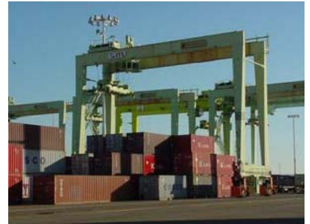
Figure 1 – Rubber Tired Gantry Crane (RTG)
